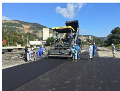
Fig.2 ISO road surface construction status
