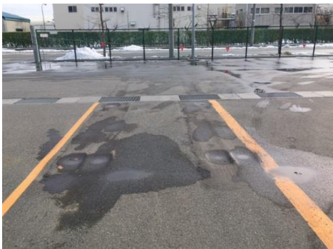
Figure-10 Condition before construction
