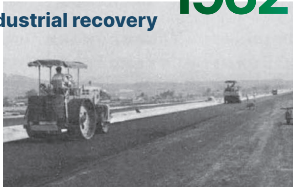
Pavement construction for Suita-Ibaraki area of Meishin Expressway
