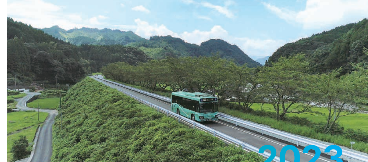
Dedicated BRT road constructed with PET Ascon
