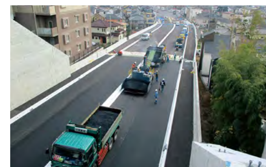
Constructed the first dual-layer noise reduction pavement in Saitama Prefecture
