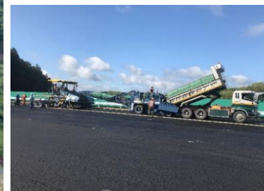
Deploying vertical conveyor to improve smoothness
